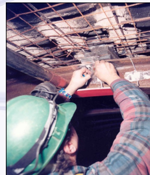
On-site Installation of a PU Encapsu- lated strain gauge
